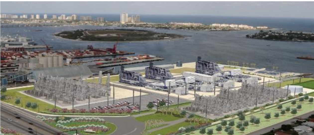
Riviera Beach Energy Center, 2014
